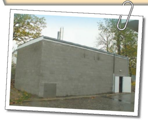
**Fuel store and fuel handling:** blockwork fuel hopper 5 x 5 x 4.5 (h) steel lid 3 x 3; hydraulic lift spring outfeeder to boiler feed screw
